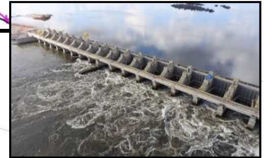
Belo Monte & Pimental Dams World's 3 rd largest hydroelectric dam
