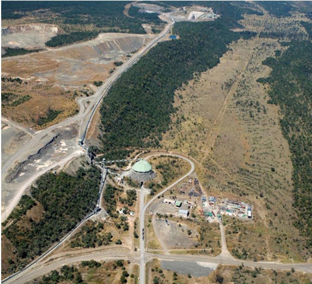
Figure 7. Aerial view of equipment and services common to Portals 1 and 2
