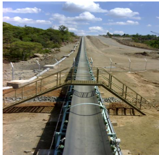
Figure 9. Portal 1 Overland conveyor
