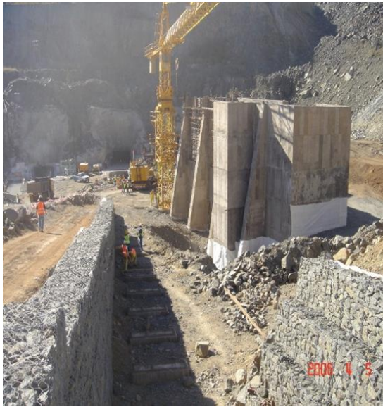
Figure 3. Portal 2 (Rukodzi) Crusher station under construction
