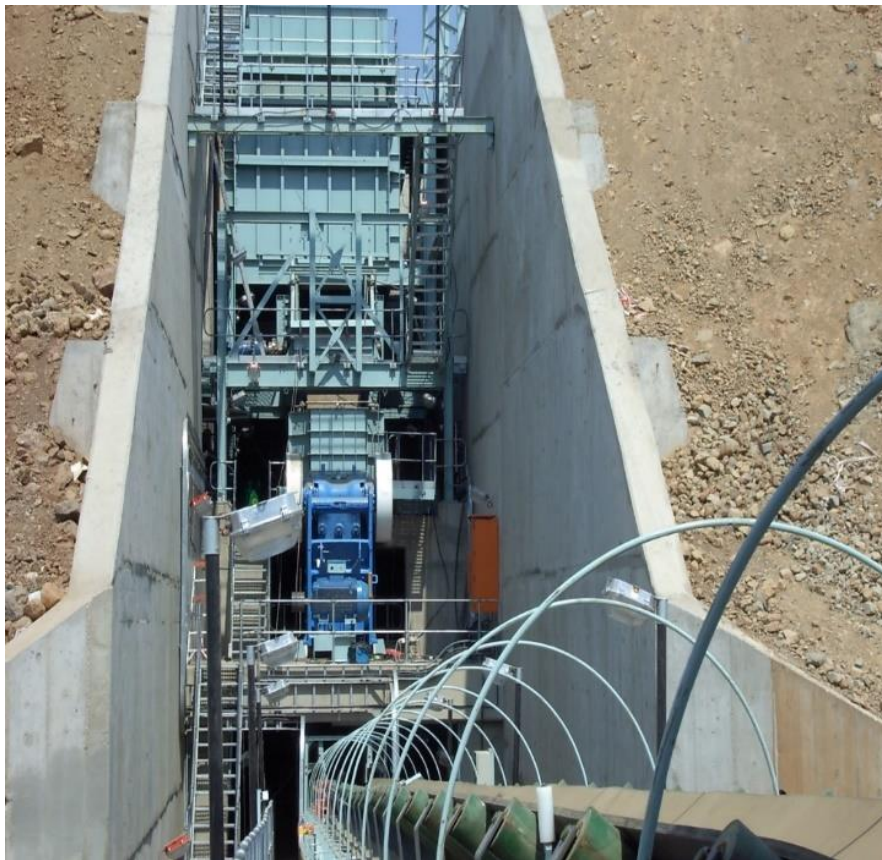
Figure 6. Portal 1 (Ngwarati) Crusher Station
