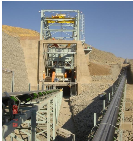
Figure 4. Portal 2 (Rukodzi) Crusher station completed
