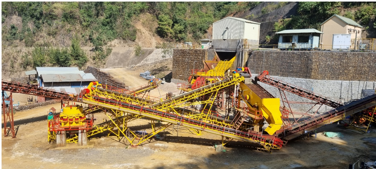
Figure 4 - Recommissioned Ban Phuc Crushing Circuit
