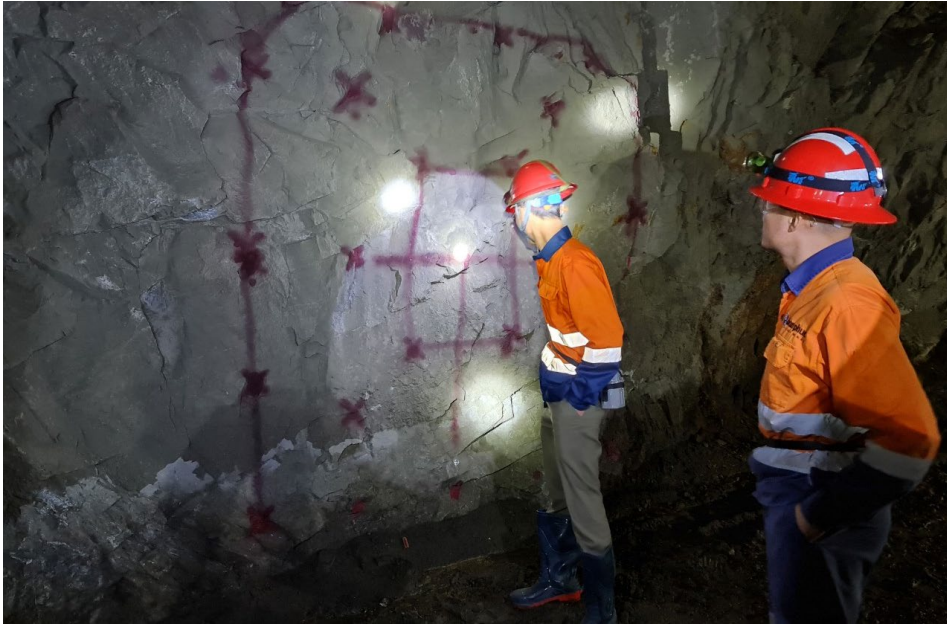
Figure 3 - First face marked out ready for drilling
