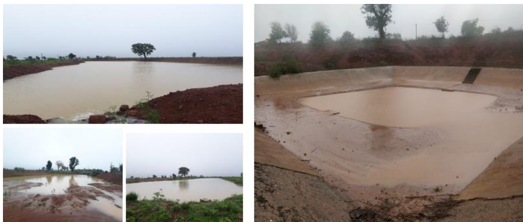
Figure 8 : Rain Water Harvesting Ponds at Bodai Daldali
