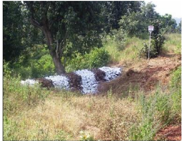
Figure 7: Check Dams Developed to mitigate run off during monsoon
