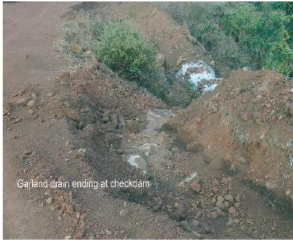
Figure 7: Check Dams Developed to mitigate run off during monsoon
