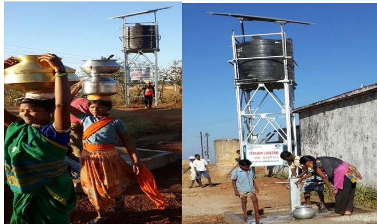
Figure 10 : Solar Powered Drinking Water Facility
