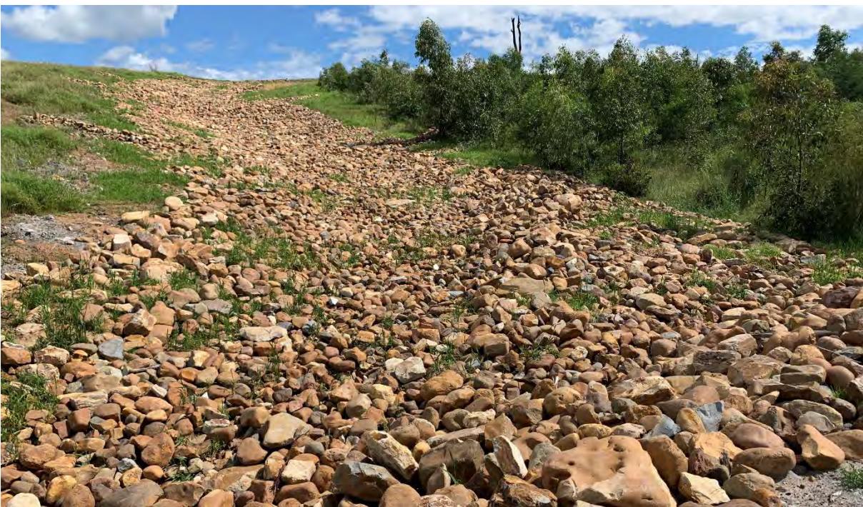
Photo 9 Natural drainage constructed within a geomorphic natural landform.
