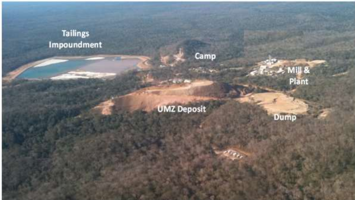
Figure 14.1: Aerial view of the Don Mario Infrastructure looking southwest
