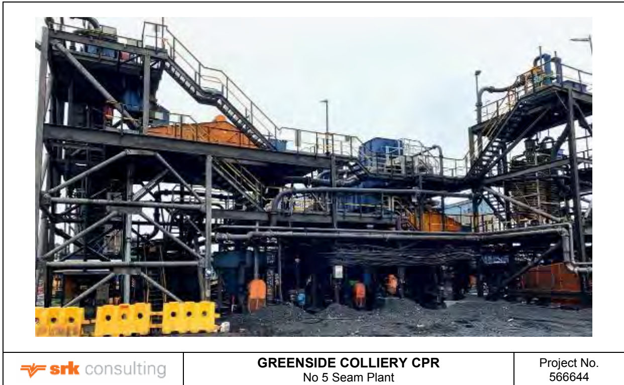
Figure 10-23: No 5 Seam Plant
