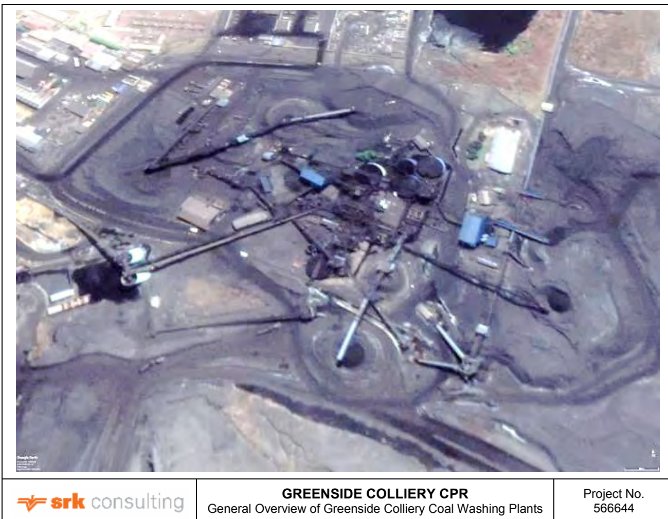
Figure 10-1: General Overview of Greenside Colliery Coal Washing Plants
