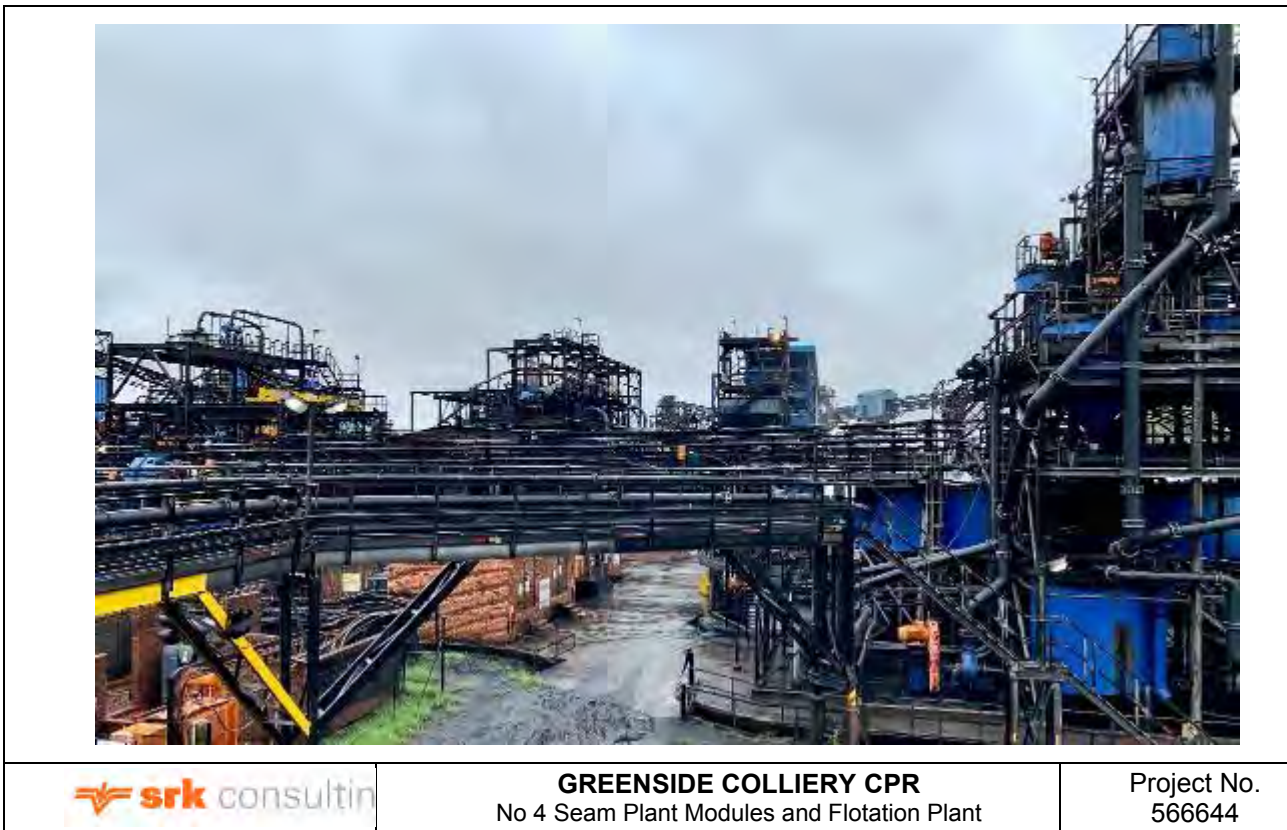
Figure 10-8: No 4 Seam Plant Modules and Flotation Plant
