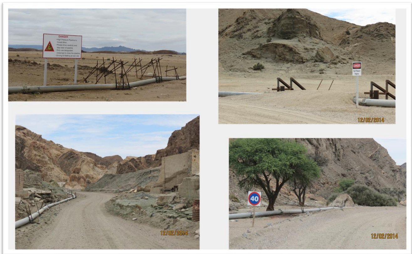
Figure 5-2: Photographs of The Pipeline Along The Khan Mine Valley Route – 2014.
