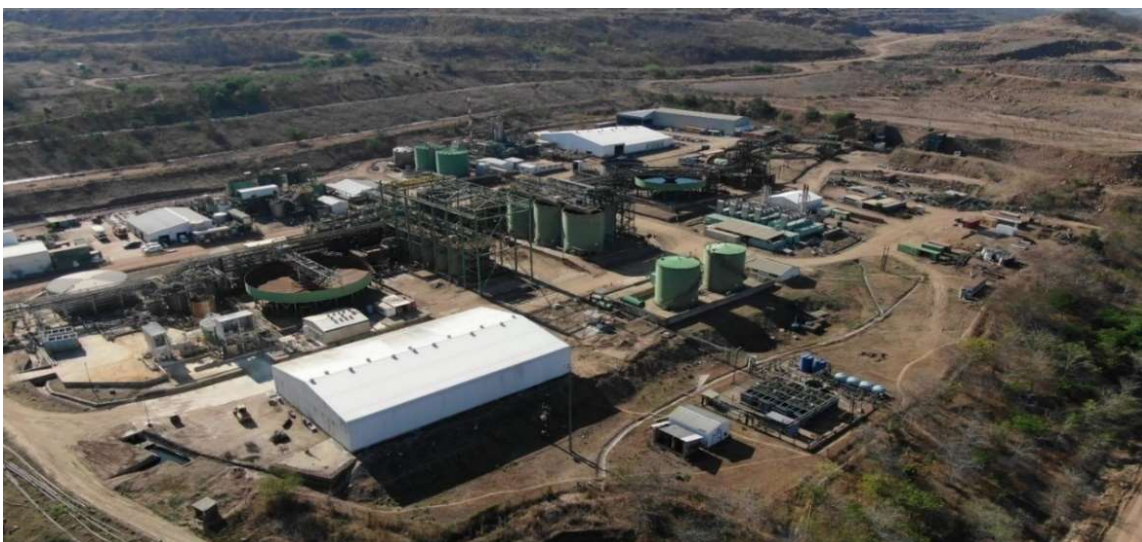
Figure 1 - Kayelekera uranium project in Malawi was in production from 2009 to 2014
