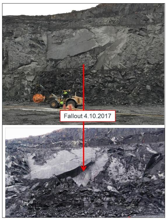
Figure 14-14: Example of typical bench scale wedge or planar failures
