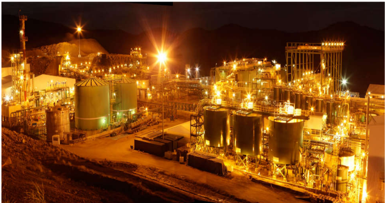
Figure 1: Kayelekera Processing Plant
