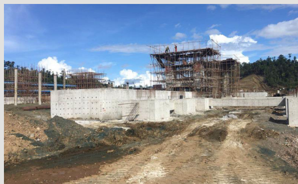
Picture taken at the RKEF Project site in May 2018.
