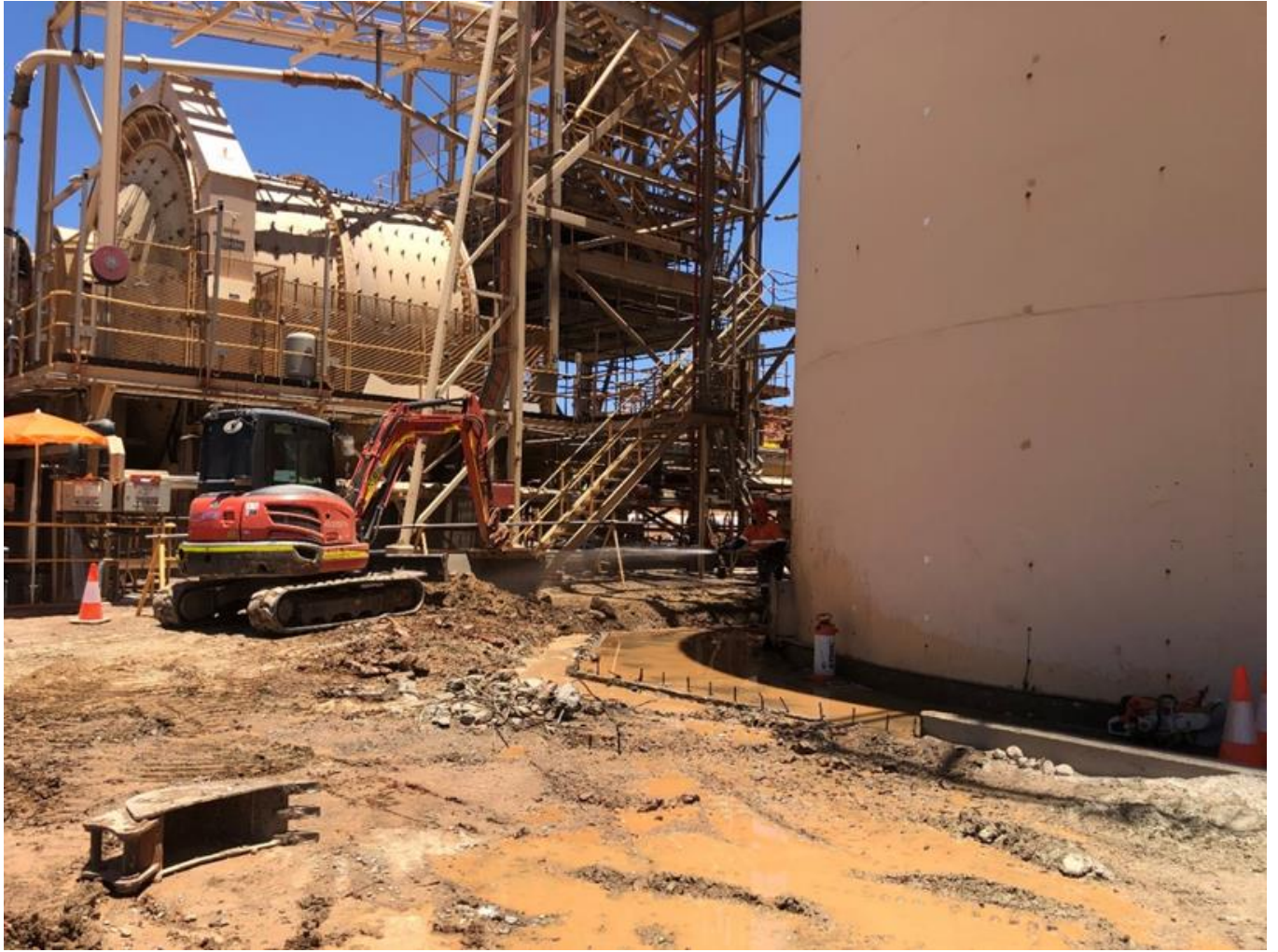
(Figure 2: Concrete repairs to the tank bund walls - view facing south.)
