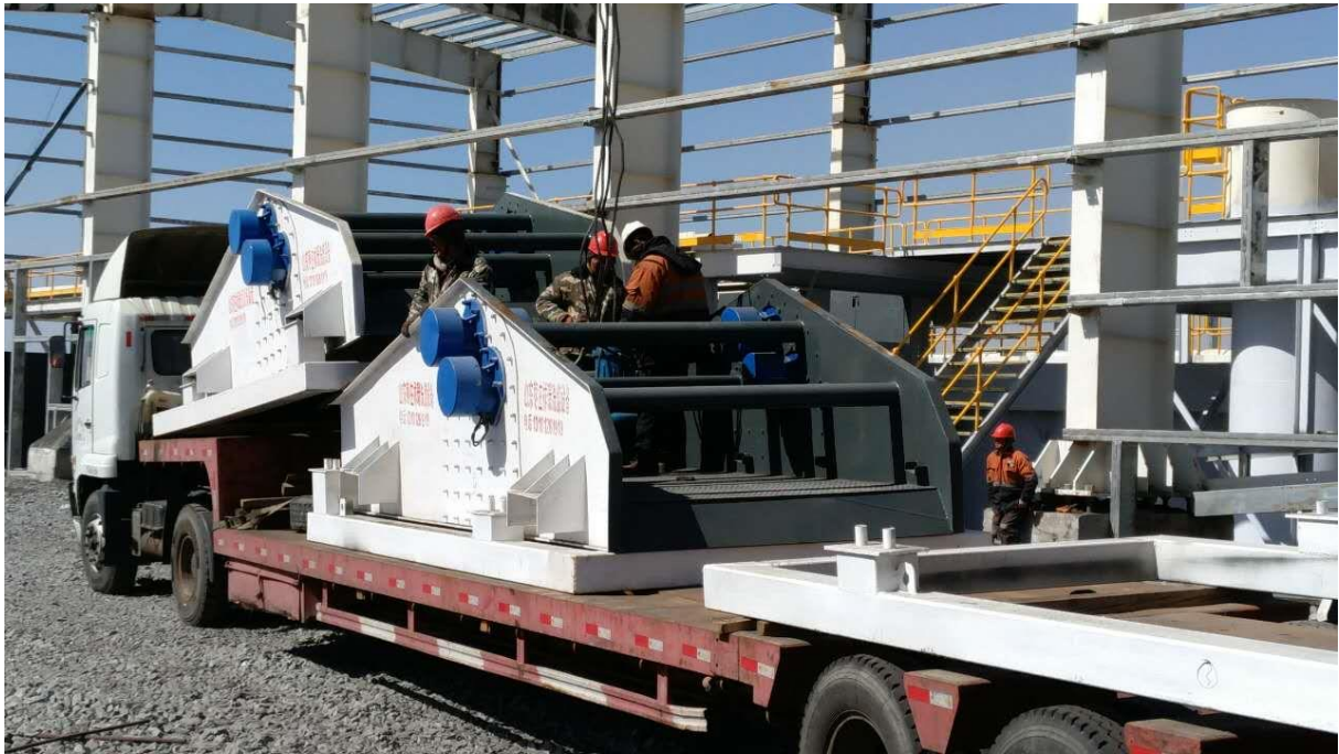
Figure 17-3: Components are delivered to the Mine Site for Assembly
