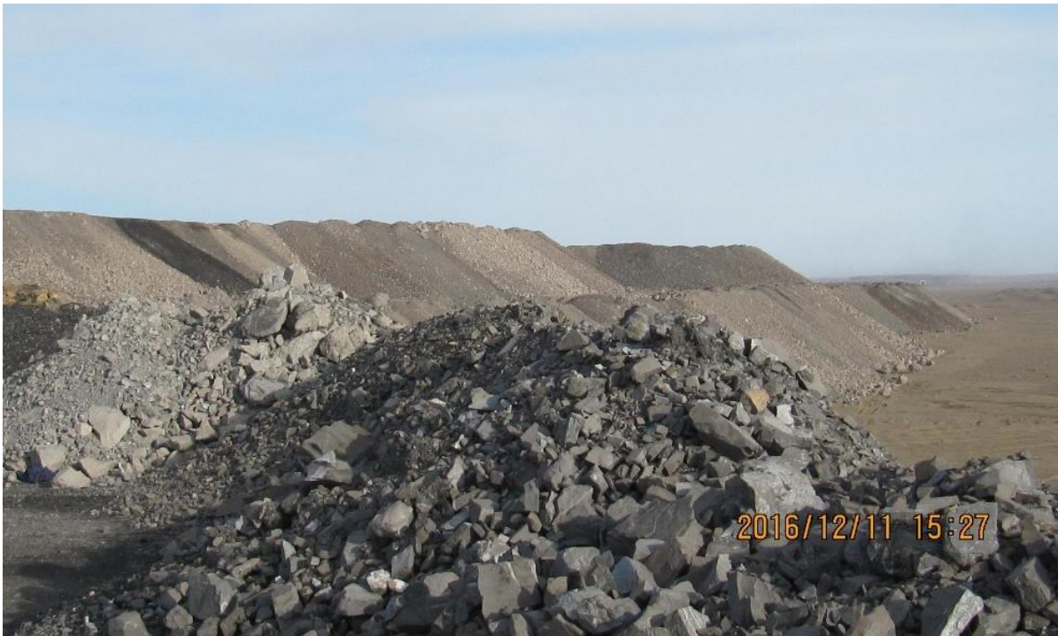
Figure 16-13: Active Ex-Pit Waste Dump of the Sunrise Pit (looking east)
