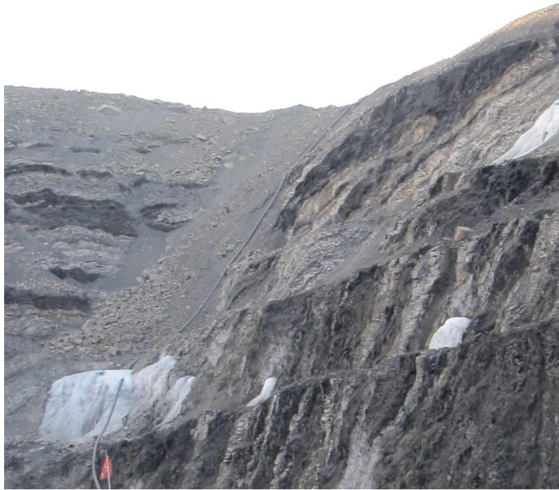
Figure 16-16: Frozen Seepage Through Pit Wall of the Sunset Pit
