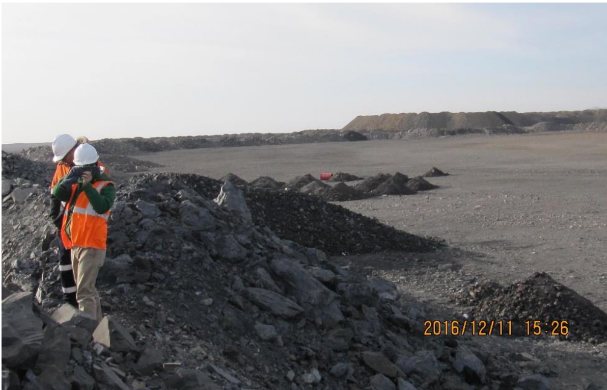
Figure 16-14: Active Ex-Pit Waste Dump of the Sunrise Pit (looking west)
