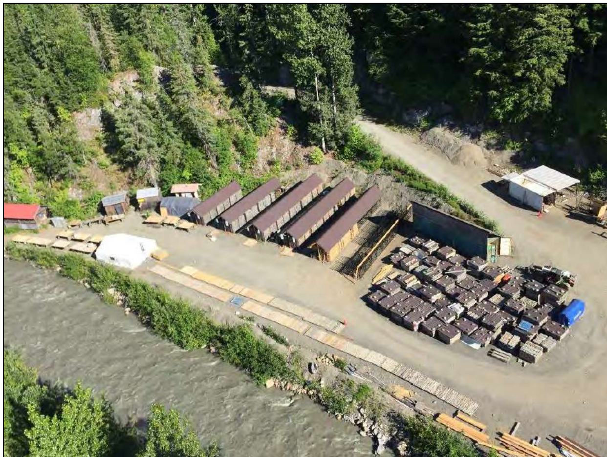
Figure 11-1: Aerial view of Porcupine Creek Exploration Camp
