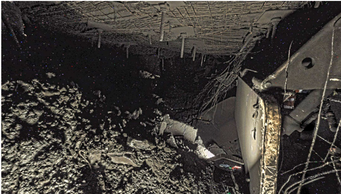
Figure 118: View into the goaf from the tailgate roadway after the serious accident
