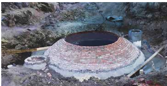
Construction of Biogas Plant at RZM Murowa
