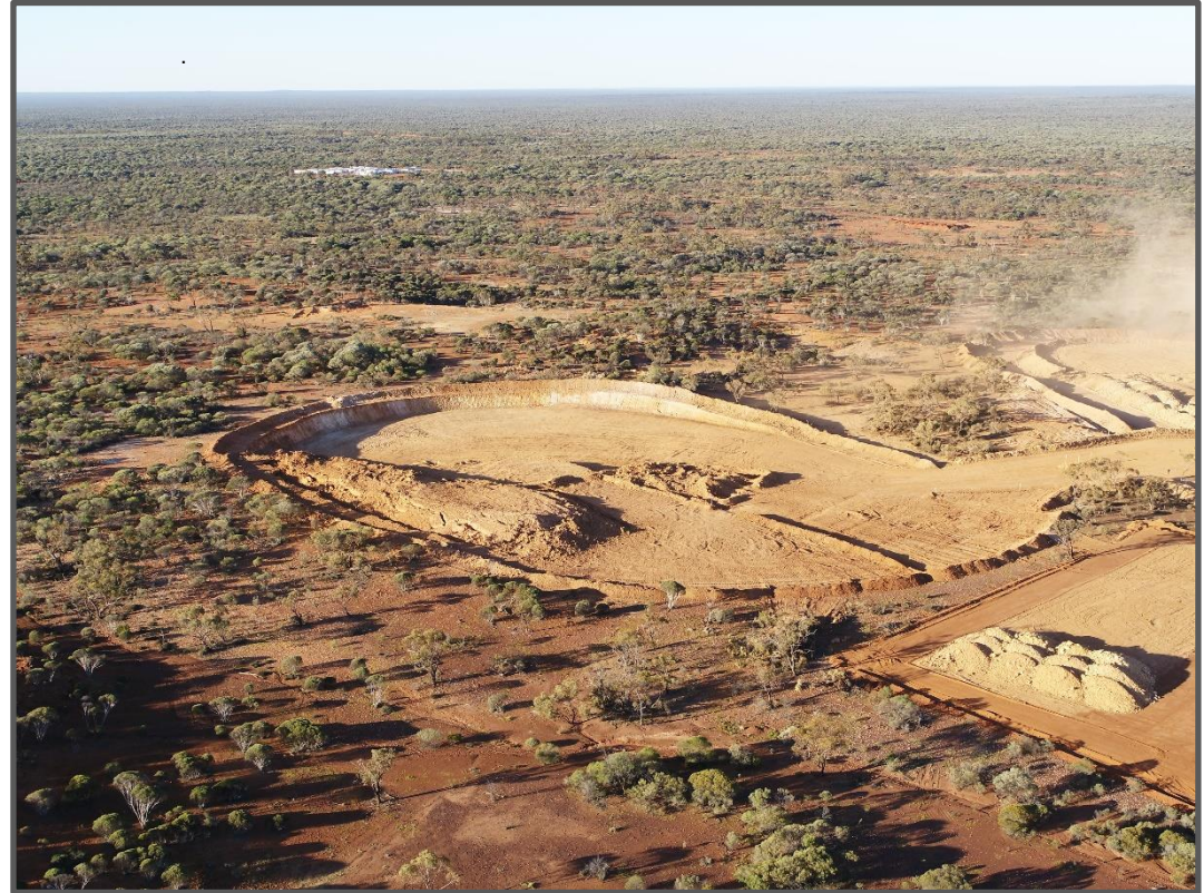
First blast complete at Magenta pit
