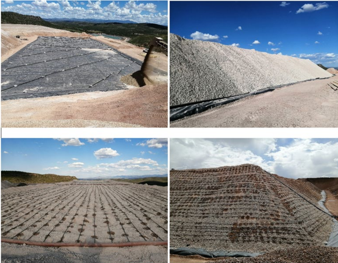
Figure 13-6: Test Heap Leach Pad Photos
