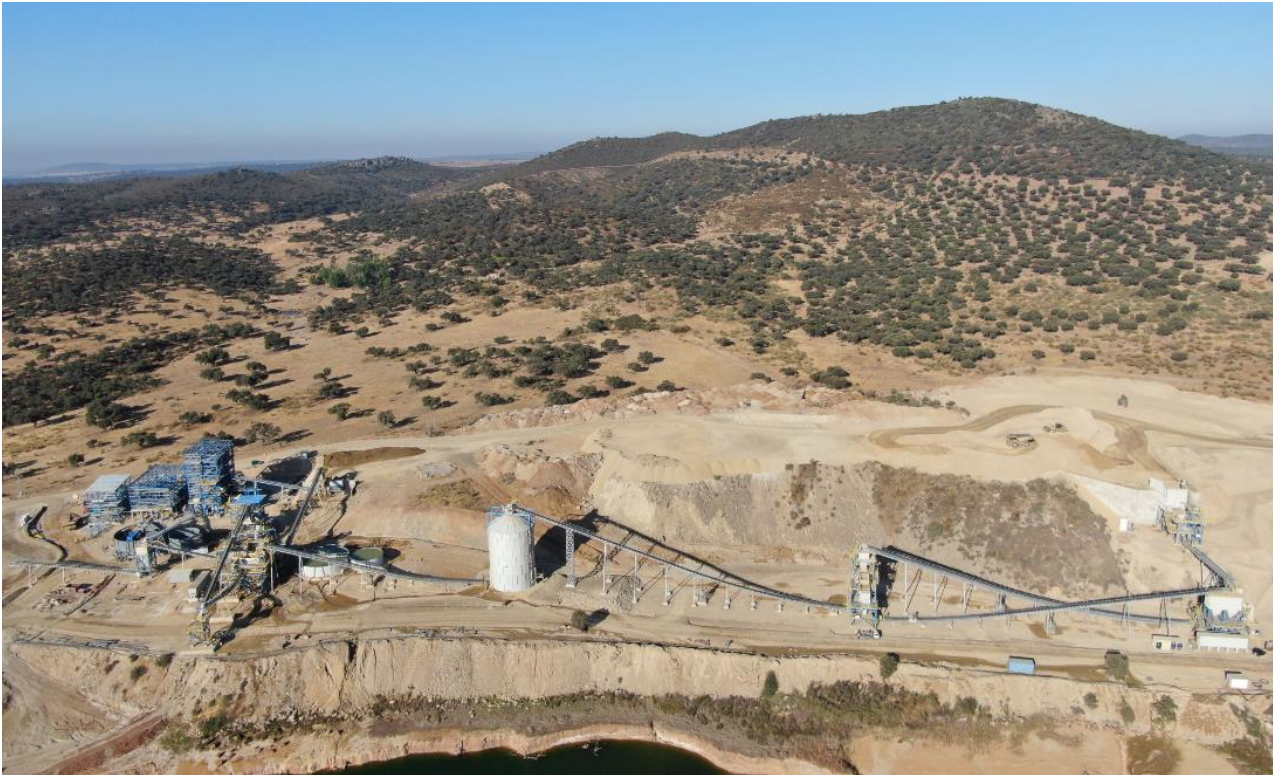
Figure 2. La Parrilla construction nears completion
