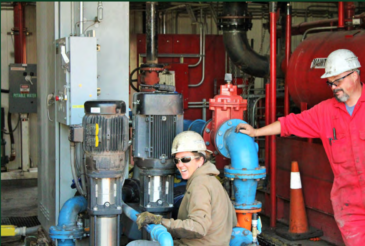
Courtni Sieler, Plant Technician and Jeremy Carnes, Electrician doing pump repairs.
