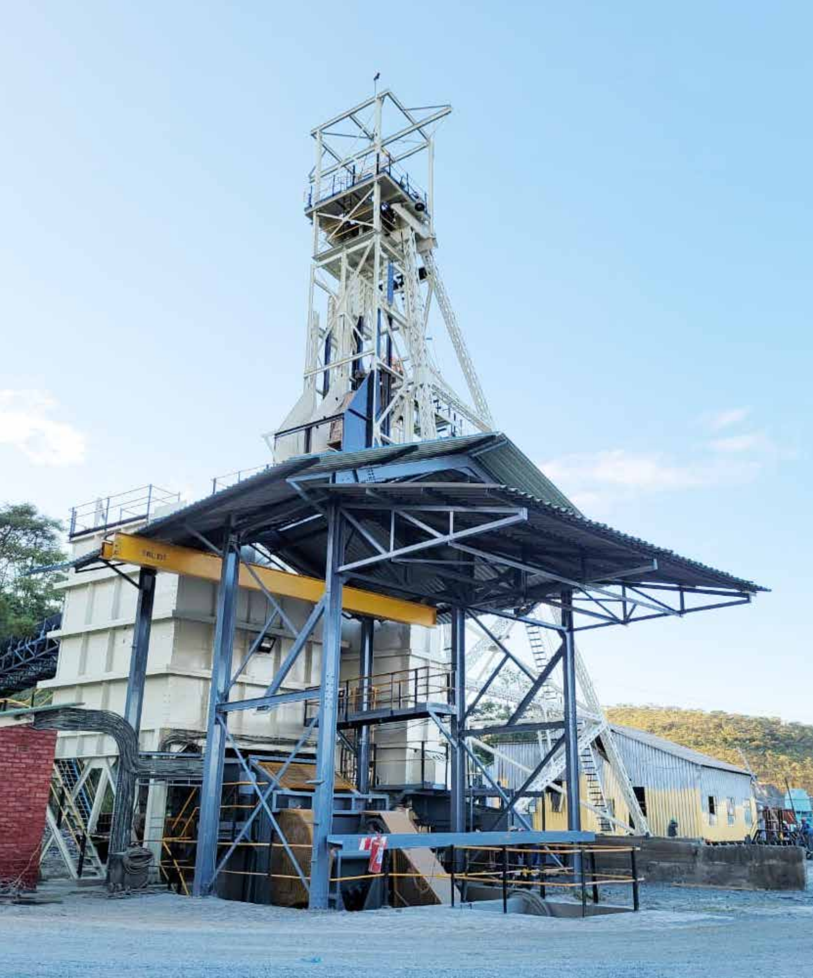
The Trojan Mine Headgear after refurbishment
