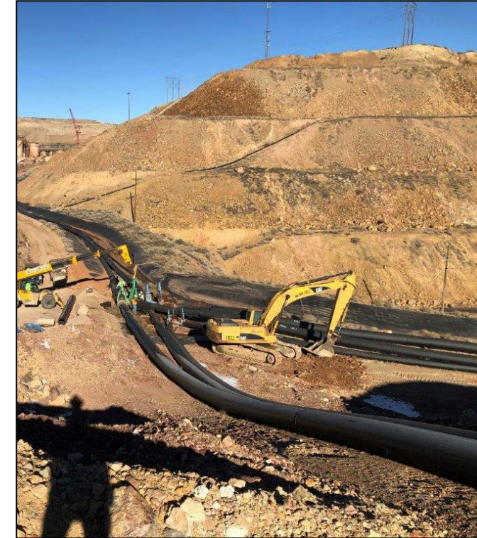
Upgraded Tails Line Installation Location
