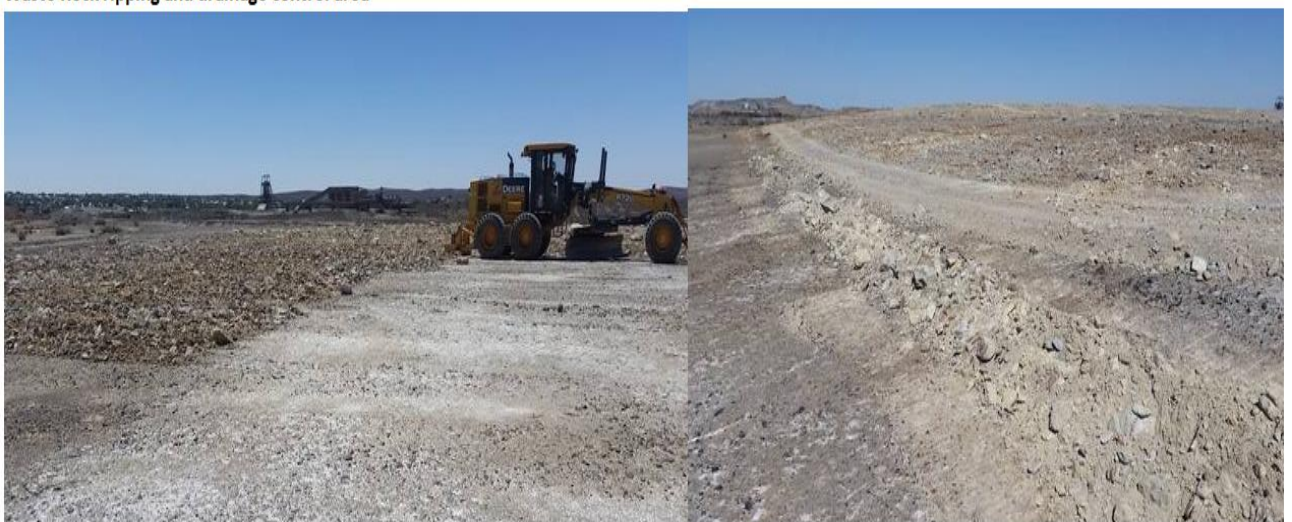
Figure 13 - Photographs of ripping and contouring activities on slime dam 1
