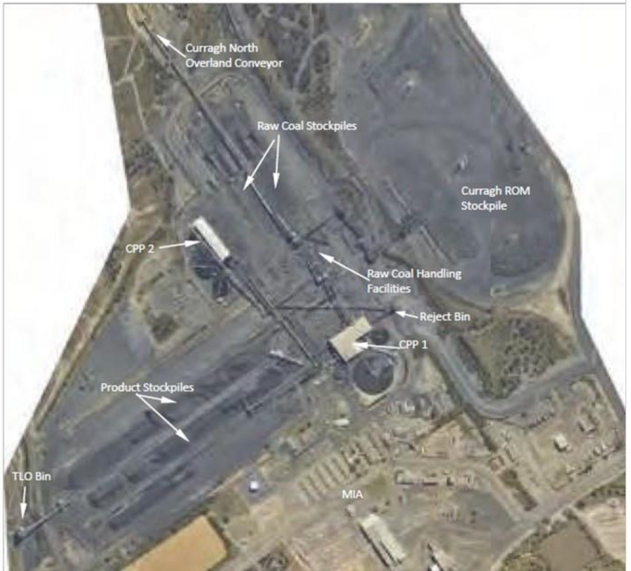
Figure 14-1: Aerial view of the CHPP facilities and associated infrastructure
