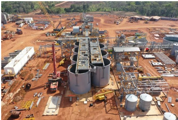
CIL top-of-tank steel platform installation
