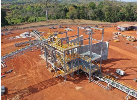
Structural steel and mechanical equipment installation in the surge bin area
