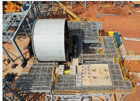
SAG mill installation
