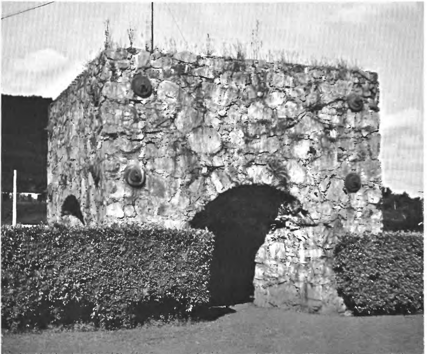
FIGURE 16.—Foundations of a blast furnace built about 1844 by Cia. Nacional de Forjas e Estaleiros at Esperança. It is reported to be the oldest blast furnace in South America. The large stone blocks were hand hewn, and the round disks on the front and side are handwrought iron washers holding tie rods that pass completely through the structure. Daily capacity was 4 metric tons.
