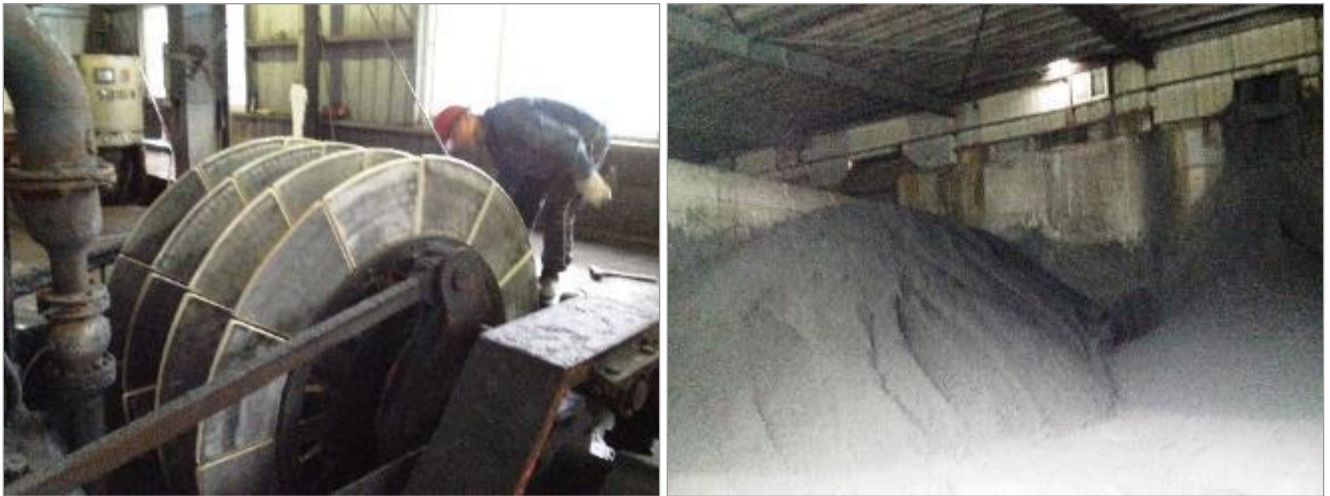
Figure 17.7 Disc filters and zinc concentrate shed
