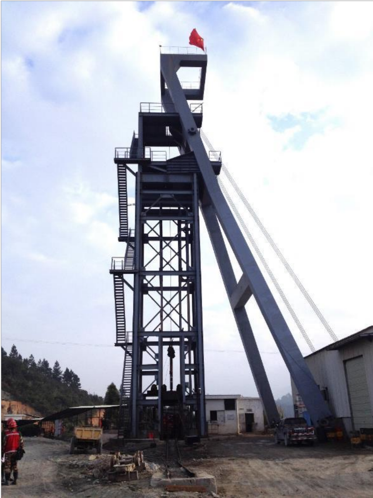
Figure 16.10 Main shaft headframe
