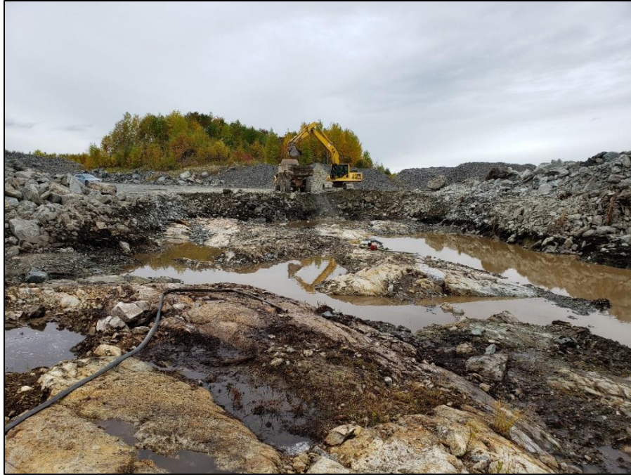
Figure 9-6 2019-2020 Stripping on Granada Property
