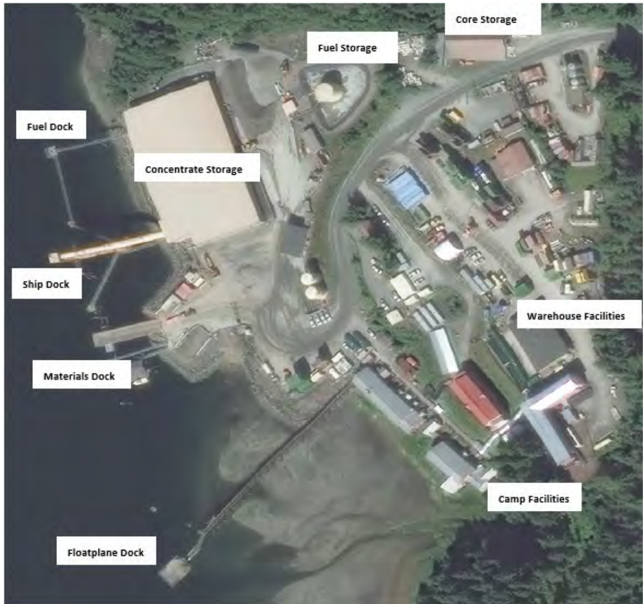
Figure 15-2: Hawk Inlet Infrastructure
