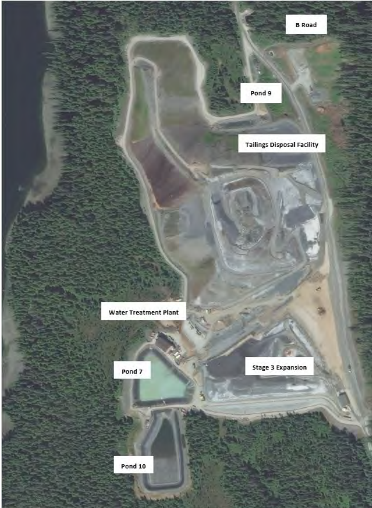
Figure 15-6: Hawk Inlet Dry Stack Tailings Disposal Facility
