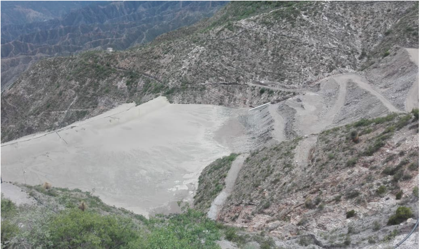
Figure 18.3 View of TSF5A (Looking Southwest - June 2021)
