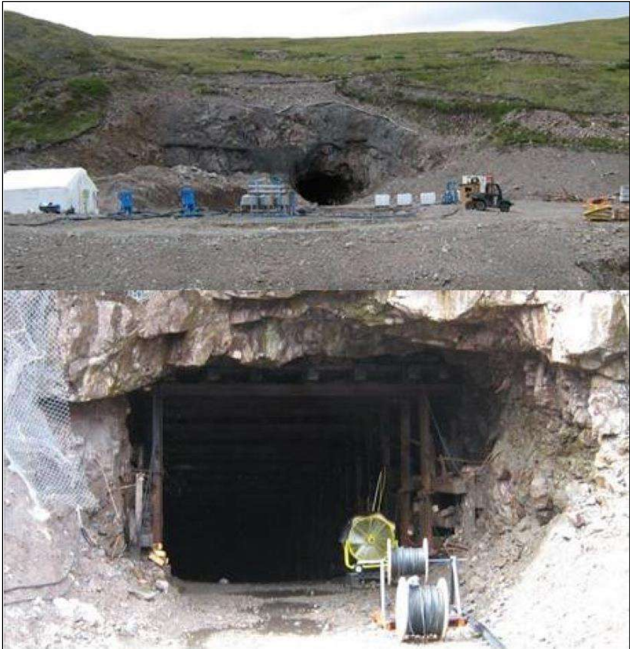
Figure 6-5: The Dewatered Cliff Creek North Portal IN 2011
