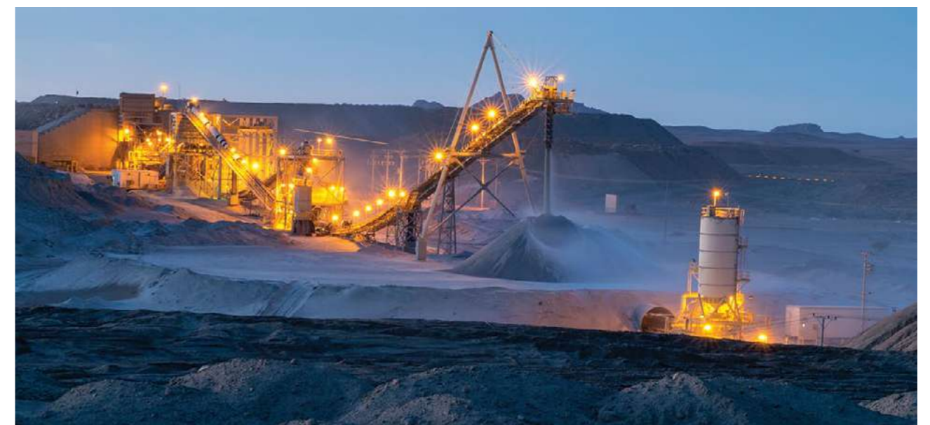
Ma'aden Gold Plant - Balgha
