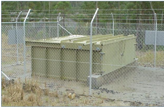
Plate 3-4 – Typical Service Borehole Site
