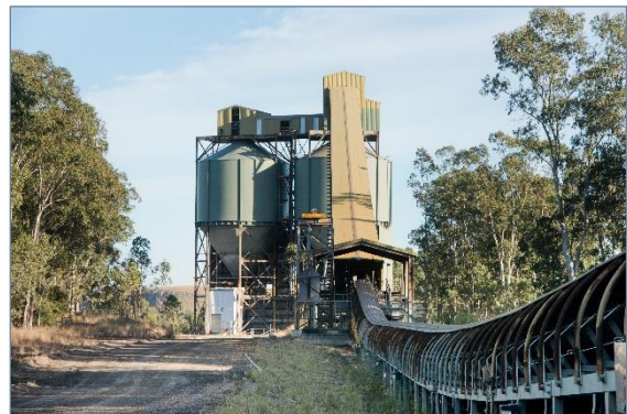
Plate 3-3 – Existing Train Load-out Facility
