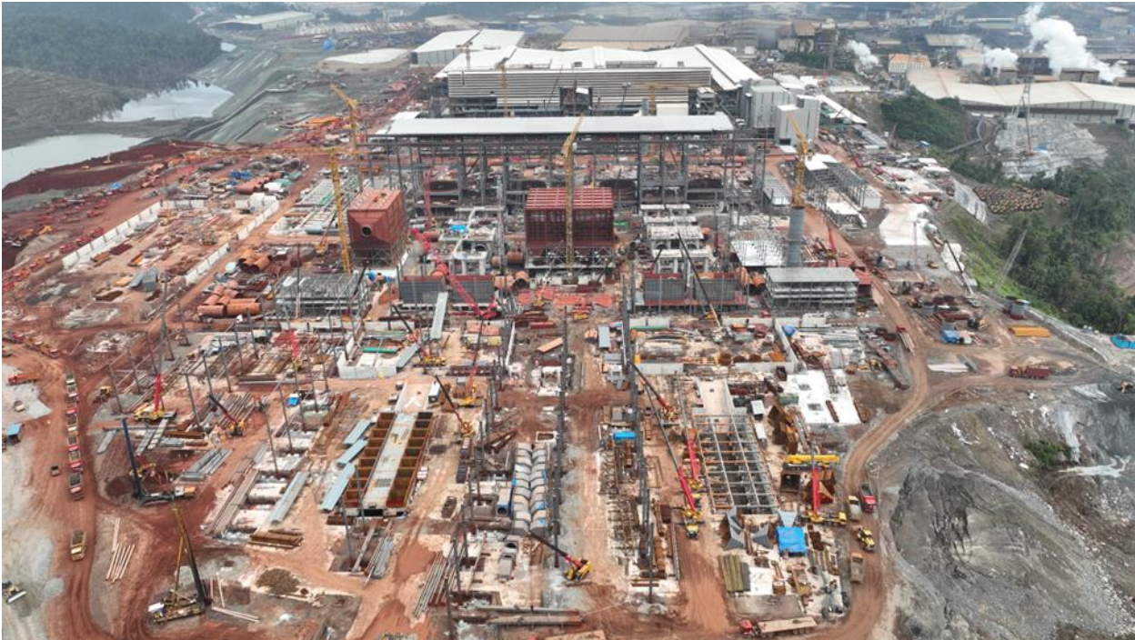
Figure 6: ZHN RKEF construction progress
