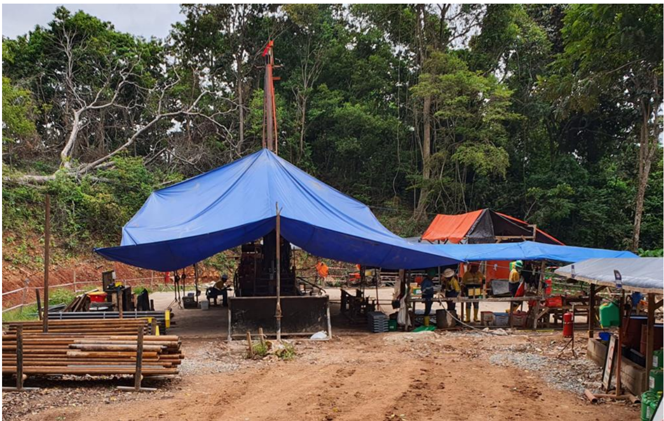
Figure 12: Diamond drilling to the north-west of Pit C
