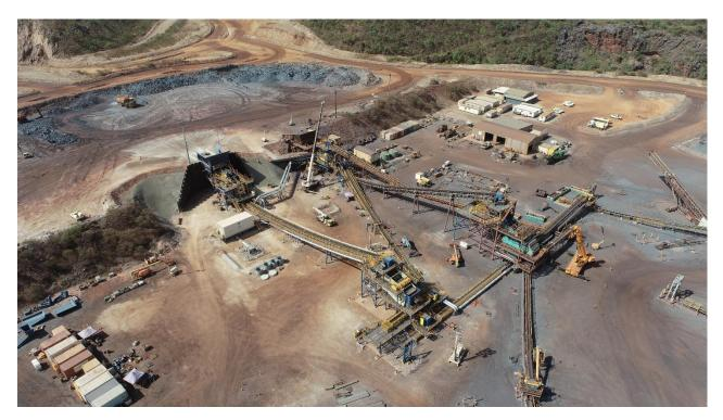
Figure 1: The upgraded Koolan Island crushing facility, showing the new ROM ore retaining wall, feed bin, jaw and cone crushers and screening circuits, December 2021.
