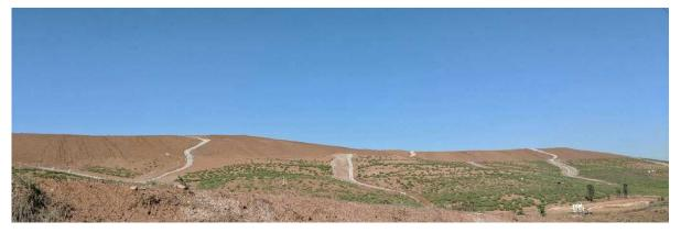
Figure 8: Re-worked contour drains on VD5
