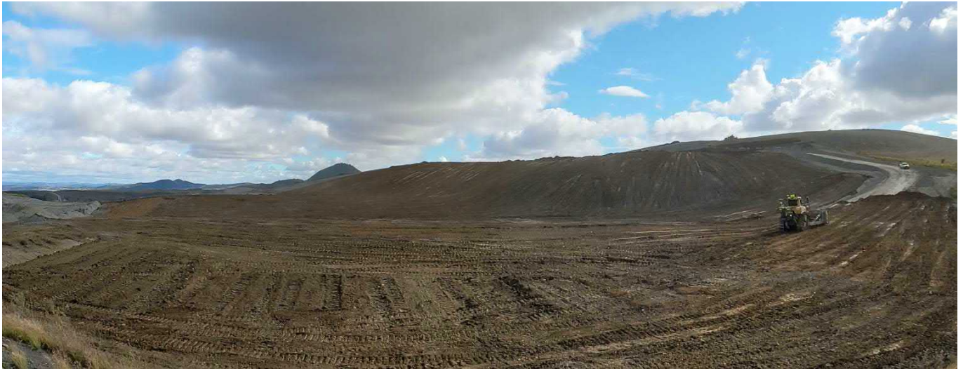
Figure 6: Topsoil spreading at Drayton Void emplacement
