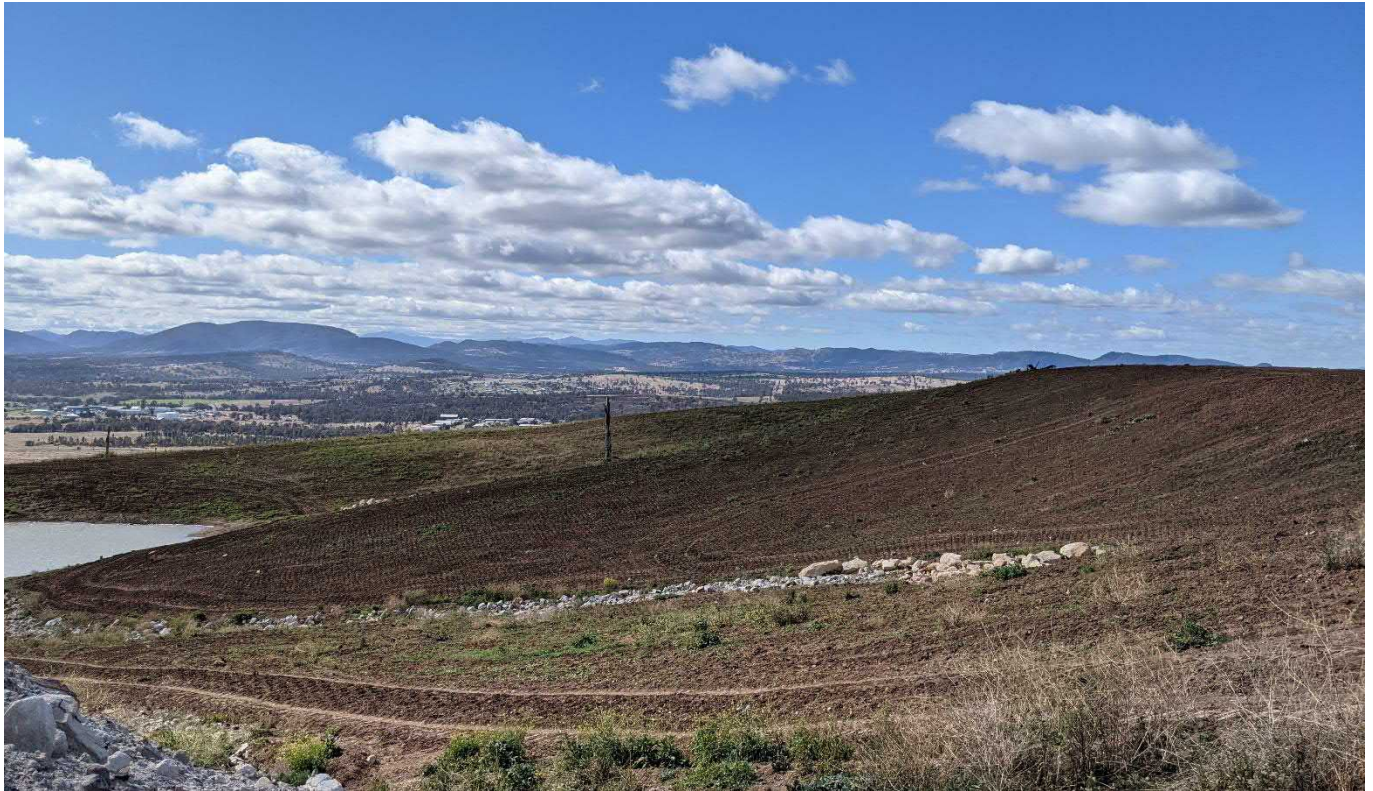
Figure 9 VD4 following maintenance work looking east
