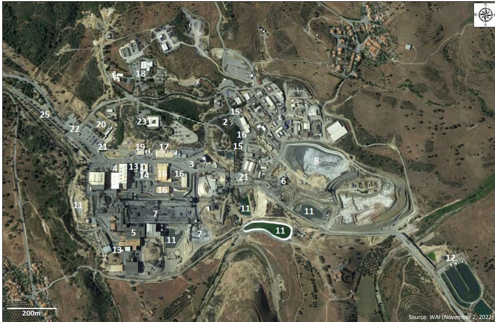
Figure 18.2: Neves-Corvo Mine Infrastructure (Inset of Figure 18.1)
