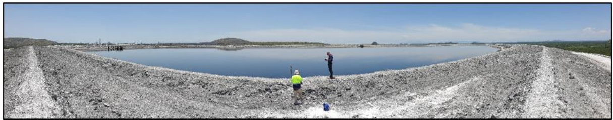
Figure 5.3: Top of stack A (looking approx. SE)
