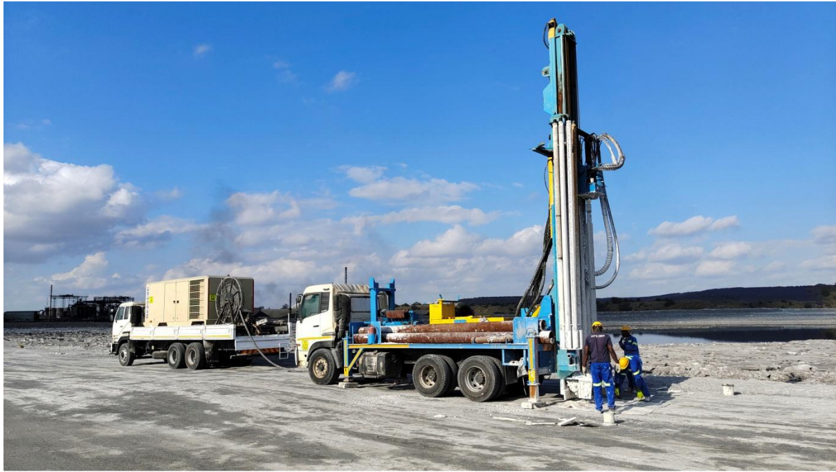
Figure 5.10: Open hole percussion rig used in the June 2022 drilling program
