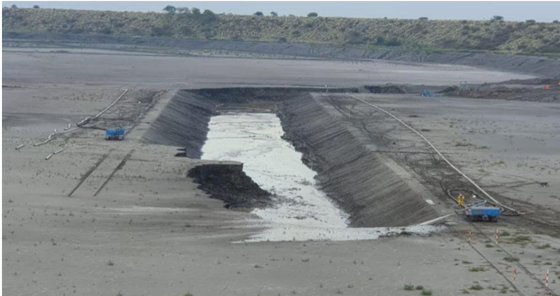
Figure 6.4: A Slimes Transport Gully Being Created Within a Residue Storage Facility
