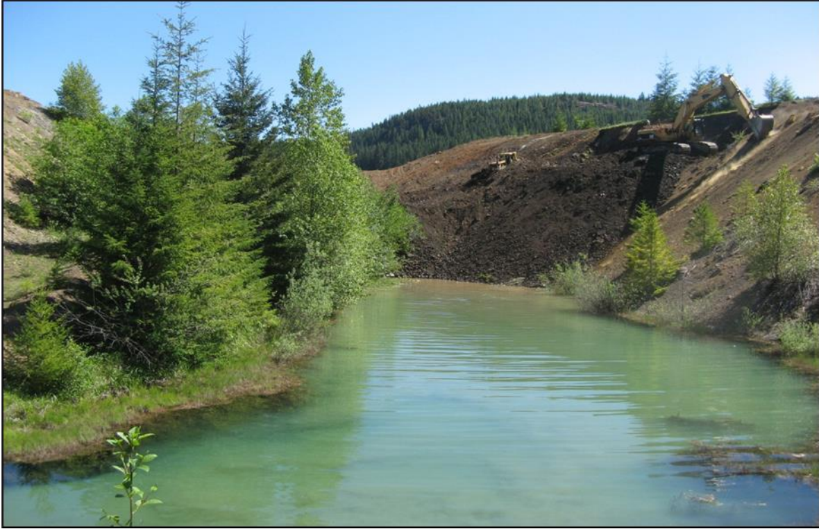
Figure 9: 1-South Sump, taken prior to the commencement of infilling 2015
