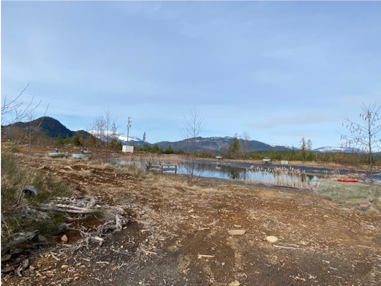
Figure 23: Sulphide Polishing Cell Passive Treatment System
