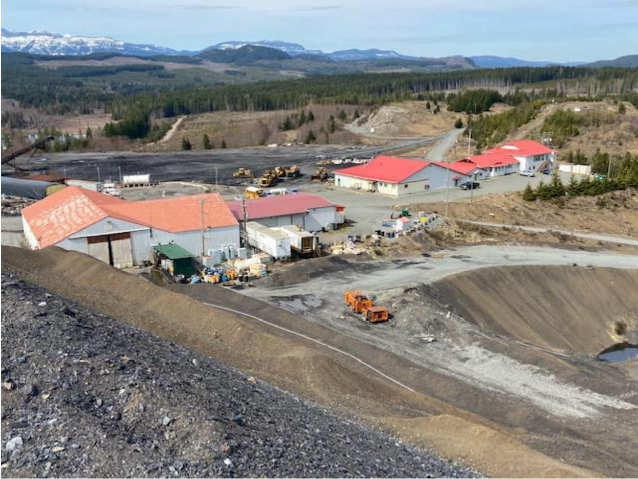
Figure 28: Administration buildings and coal pad
