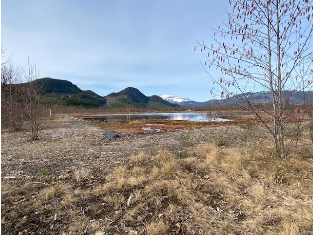
Figure 22: Biochemical Reactor, Passive Treatment System
