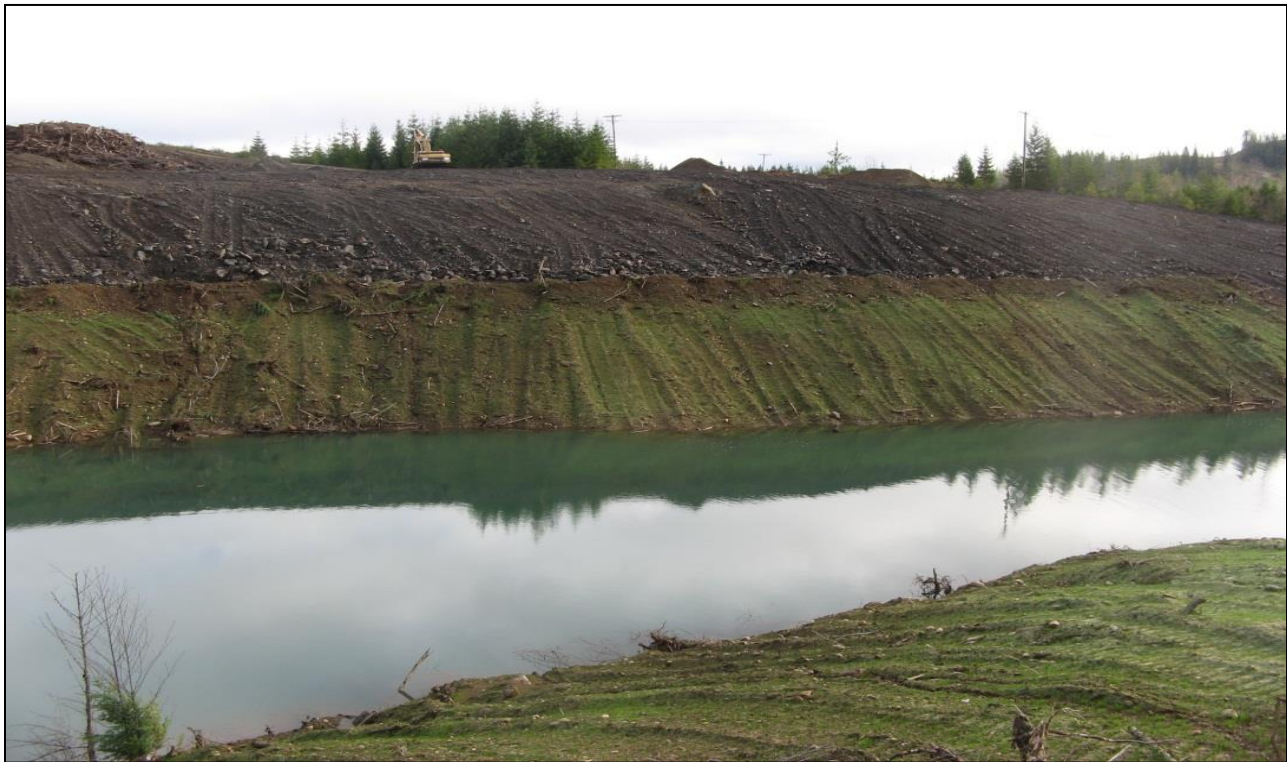
Figure 18: 3-South Pit Highwall - re-sloped, and partially revegetated, fall 2016
