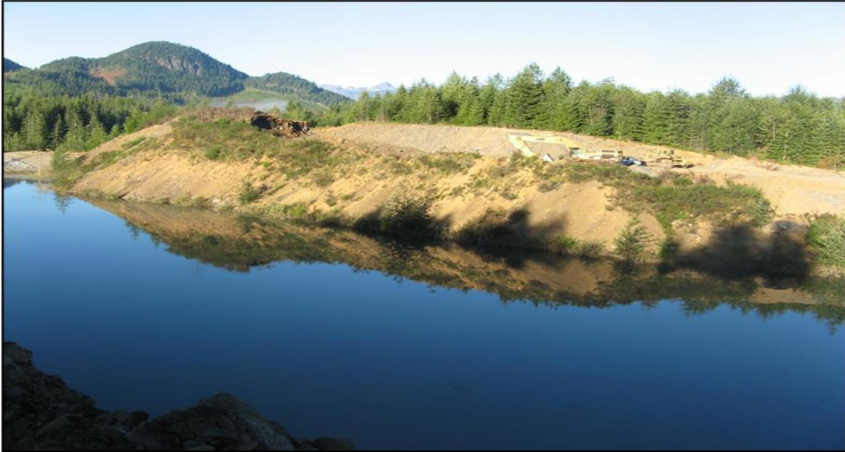
Figure 14: 3-South Pit Pond PAG-CCR Facility, looking over the North Dump area prior to reclamation
