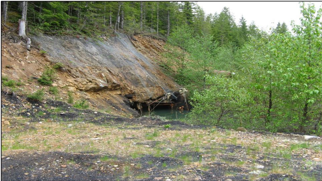
Figure 1: 242 Exploration Adit, prior to reclamation
