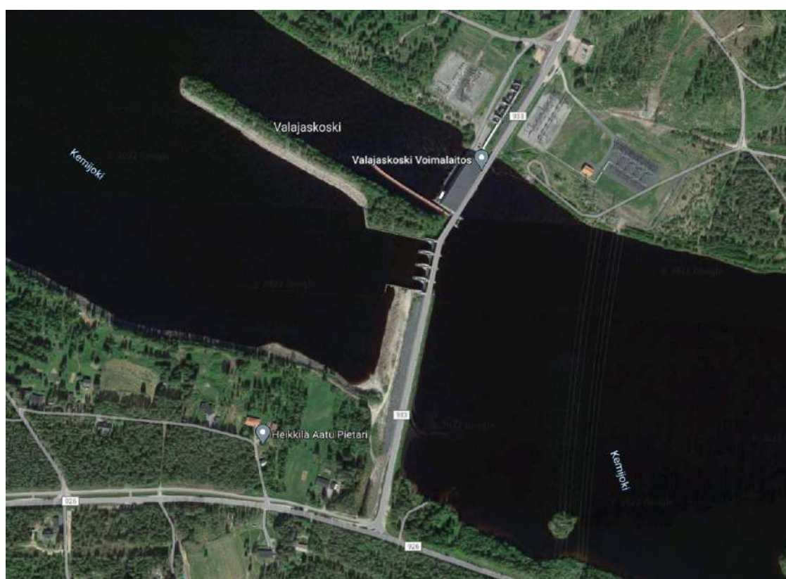
Figure 18-4: Valajaskoski hydroelectric power station
