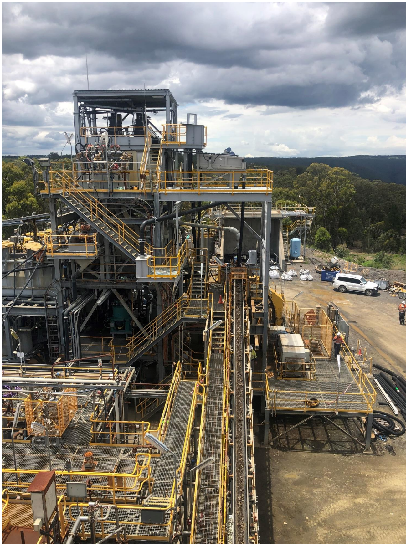
Figure 5 Ore being fed into ball mill
