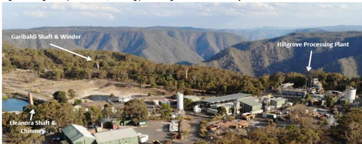
Figure 8. Hillgrove Operation Site, showing processing infrastructure and layout
