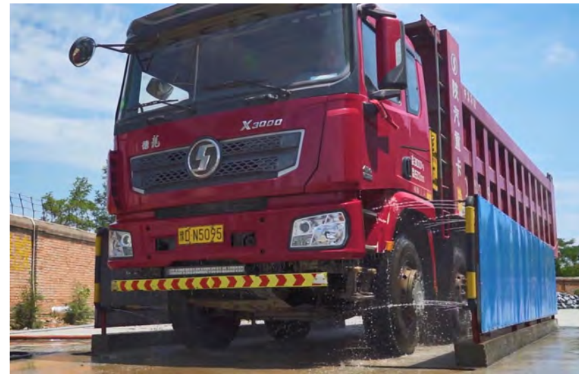
Truck flushing to reduce dust carry
