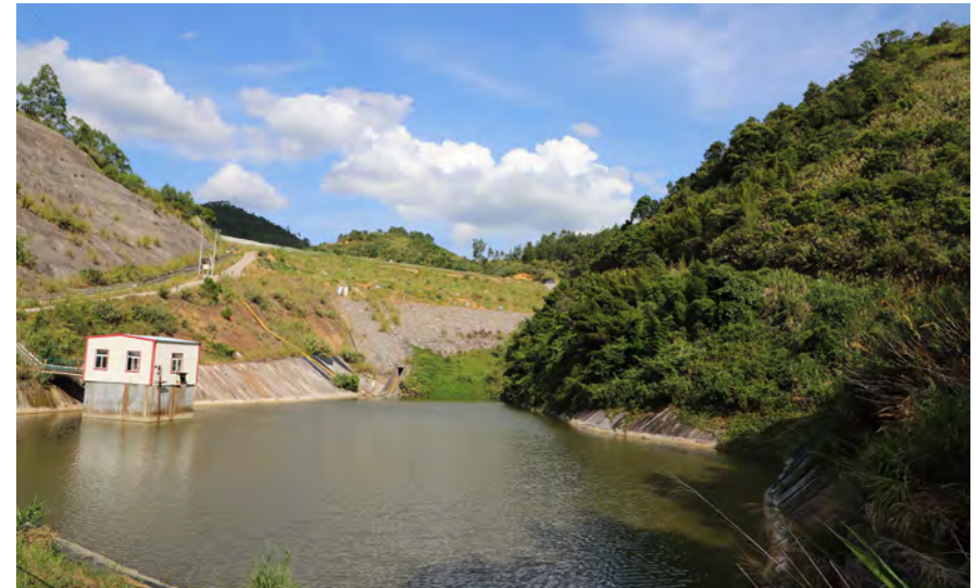
Rainwater and process water diversion system at the GC mine
