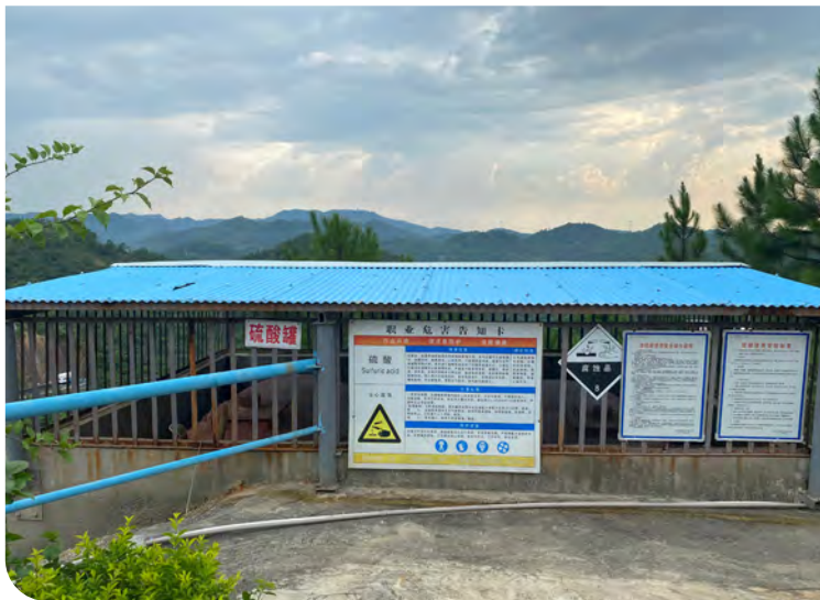
Nitric acid storage area
