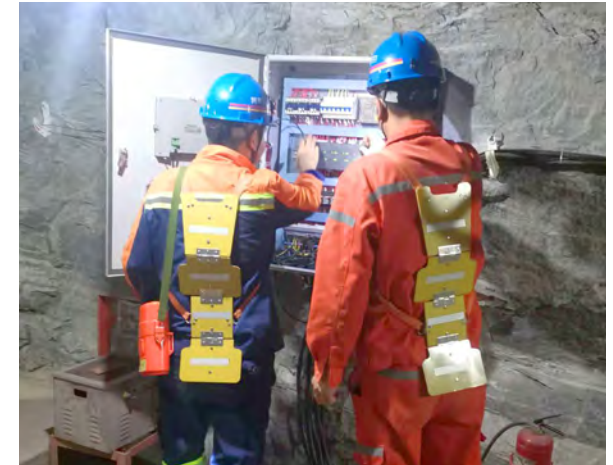
Electromechanics Department of the TLP Mine upgrades the main pumping station with the automatic control system
