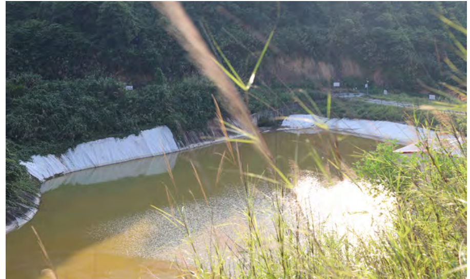
TMF anti-seepage reinforcement and dam regreening
