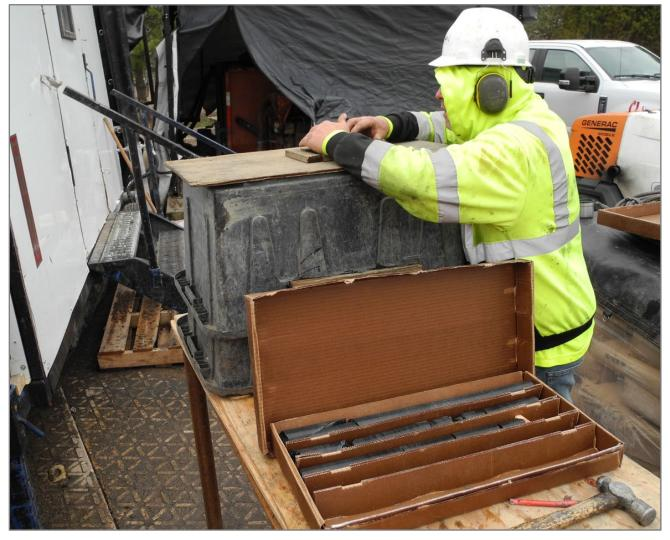
The collection of the drill cuttings into weather sheltered bins (Figure 12.9), and the subsequent disposal of the cuttings, was discussed with the drill supervisor. The drill supervisor stated that the State of Minnesota had quite high standards for environmental protection, and the drilling activities had been routinely visited and reviewed by State regulators.
