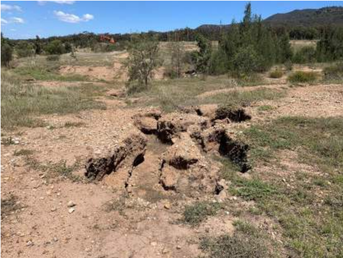
Photograph 18: Gully erosion within the North Wambo Creek Diversion (near site 23R) in 2021
