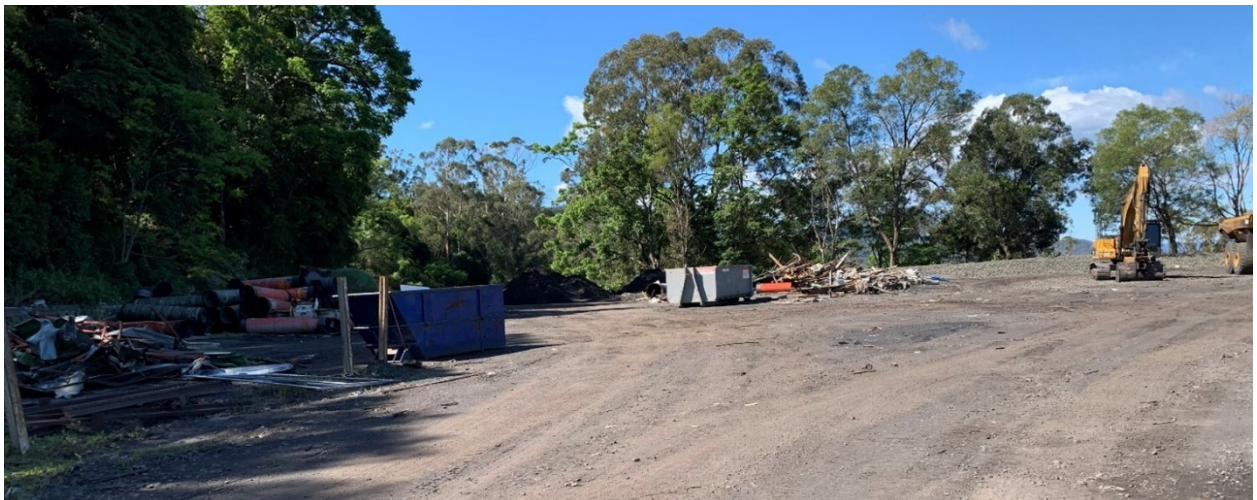
Figure 5.1: Timber Yard 8 October 2020
