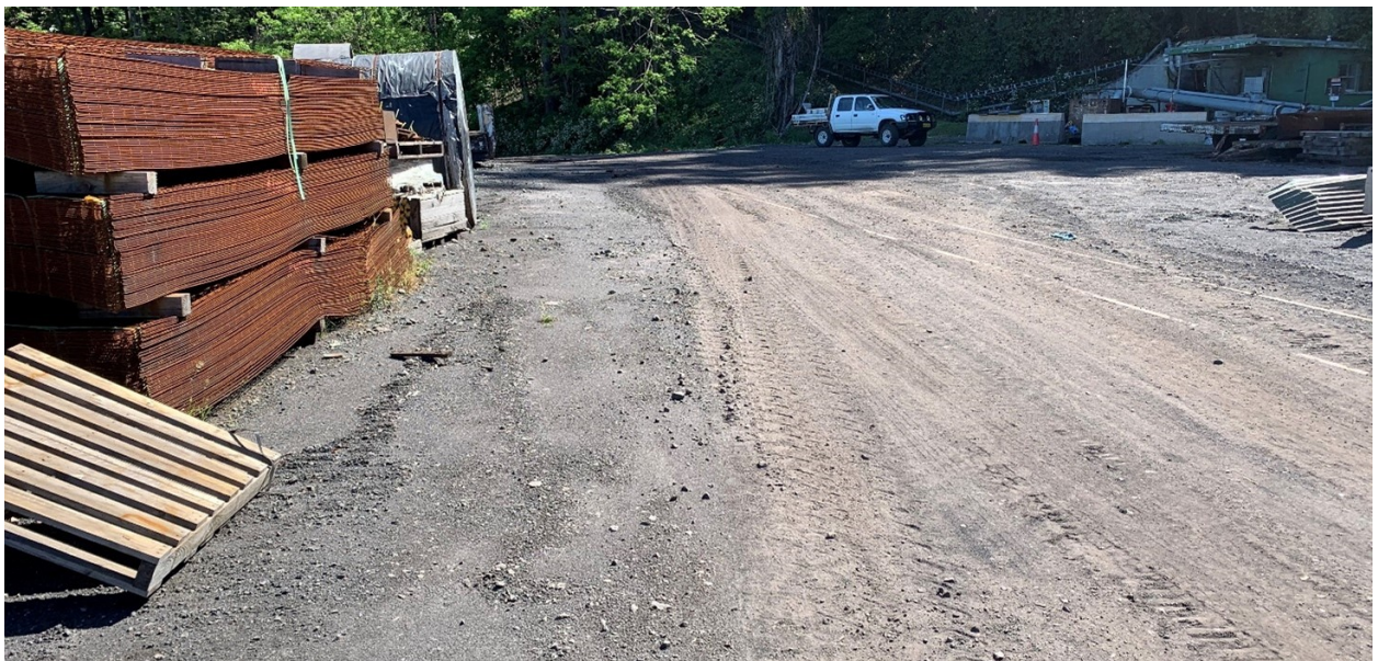
Figure 5.2: Timber Yard 8 October 2020
