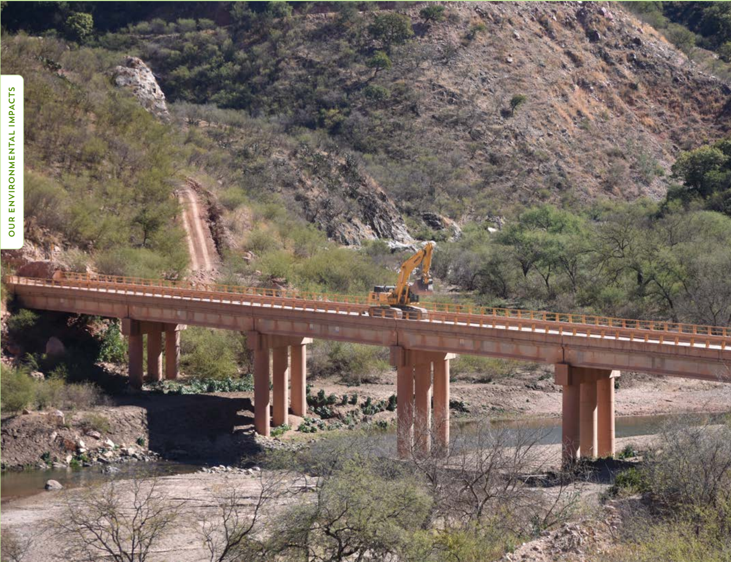
An excavator crossing the Mulatos River at the Mulatos mine, Mexico.
