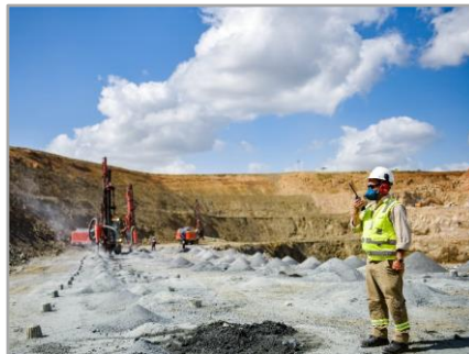
Serrote pit drilling
